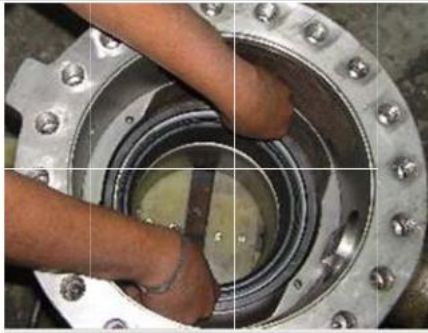
Fig.9. Seat ring assembly inserted into the body
